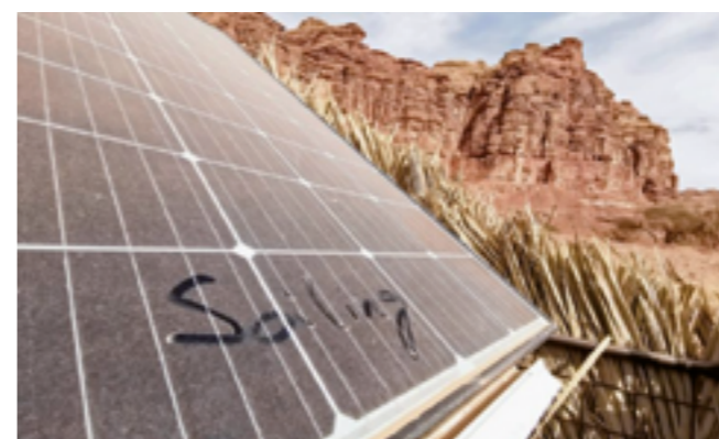
If grime is deposited on photovoltaic modules, less light reaches the solar cells and the power yield is reduced. This problem is particularly relevant for the growing use of photovoltaics in desert areas and regions with high levels of air pollution. © Fraunhofer CSP
